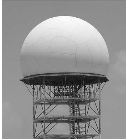
Figure 1.1 Radome-enclosed air traffic control radar antenna at an airport. (Photo courtesy of USDigiComm Corporation.)
