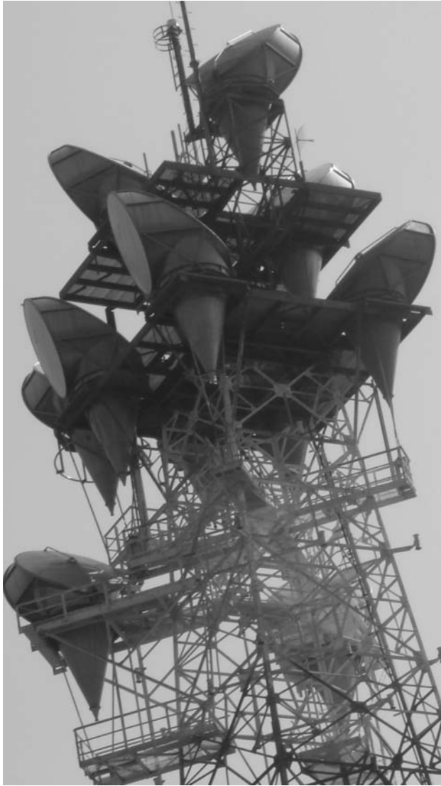
Figure 5.9 Photograph of thin wall radome covers over horn antenna apertures. (Photo courtesy of USDigiComm Corporation.)
