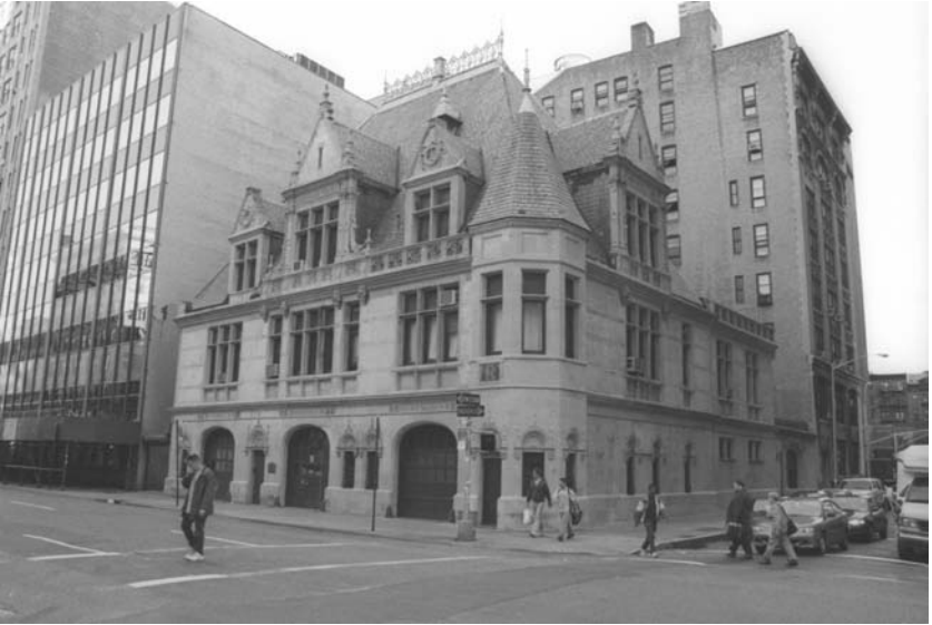
6. This landmark firehouse in New York City's Chinatown is home to Downtown Community Television. (Photo by the author)
