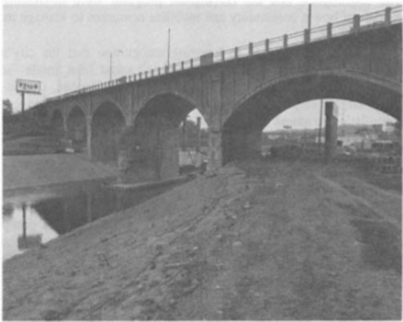
Figure 3-C Accumulated "superficial" deterioration and subsequent structural damage on Cincinnati's Ludlow Viaduct were a direct result of the neglect of maintenance, attributable to legislative budgetary decisions. Until repairs could be made, the bridge had to be closed to truck traffic, adding substantially to street congestion and the costs to businesses located in the area.
