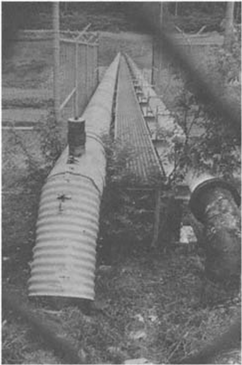
Figure 1-A Many elements of the infrastructure interact underground, hidden from view. Here water supply pipelines surface and are supported by a bridge across a concrete-lined stormwater drainage channel that replaced a creek.
