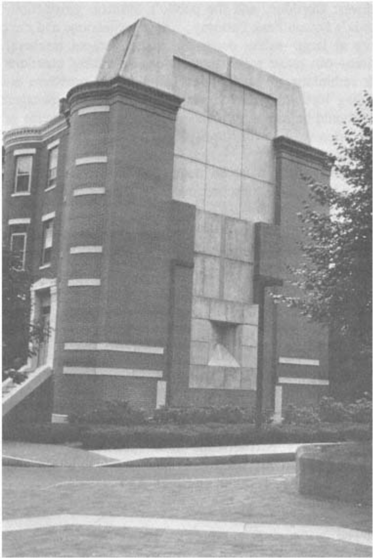
Figure 4-A In Boston's South End neighborhood, matching the design of the subway transit's ventilation tower to the style of adjacent residences converted a potential eyesore and source of community resentment to an attractive and accepted addition to the urban landscape.
