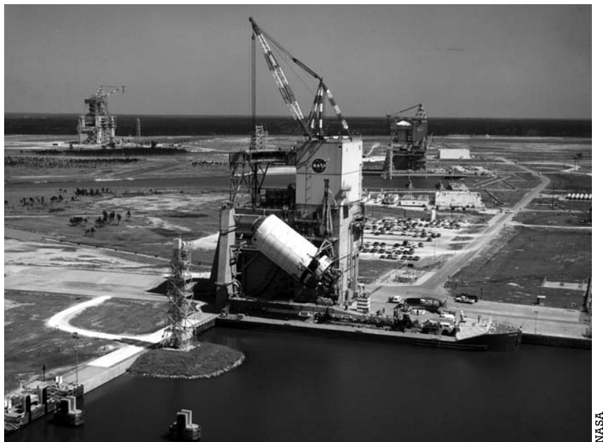
The second stage of a Saturn V rocket is lifted onto the test stand at the Stennis Space Center in 1968. Other test stands can be seen in the background. The rockets were transported by barges using the waterways.
