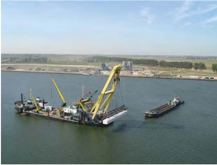
Figure 9.2. Placing of geocontainers
