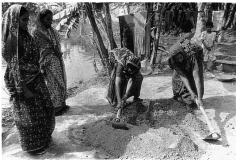
Plate 5.2 Road construction and repairs, as in Bangladesh, may be locally organised and labour intensive, but earth and gravel roads deteriorate rapidly under heavy vehicle use and may be seasonally impassable (Photo: Intermediate Technology/Neil Cooper).
