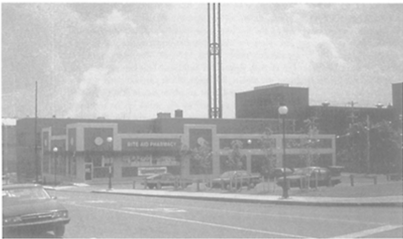
FIGURES 5.1 and 5.2 Gaspar Block, Geneva, NY, 1990, 1993. Photographs reveal the impact of new development on a city built in the nineteenth century
