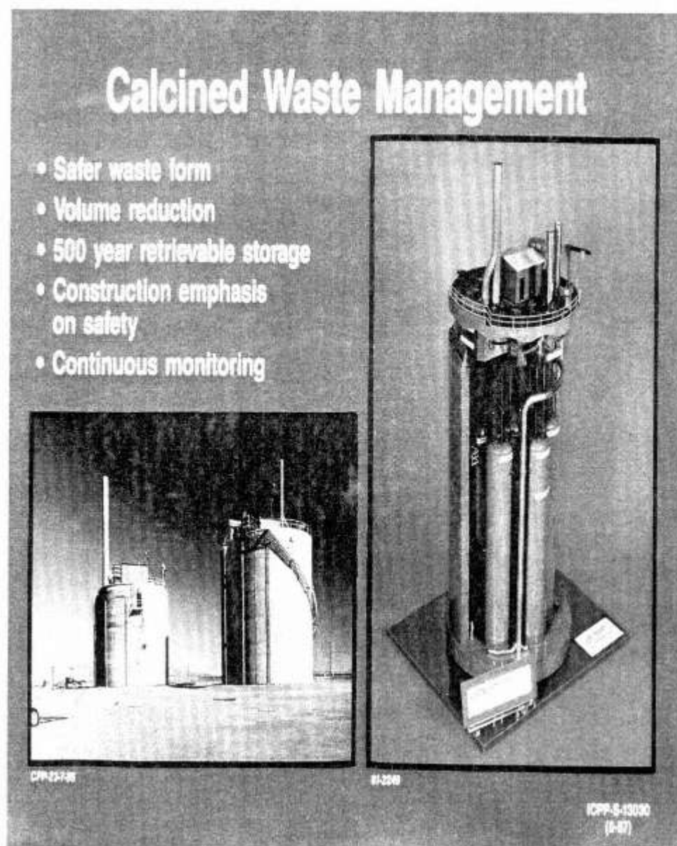
Figure 1.1(b) The photograph on the left shows Bin Set 5 and Bin Set 6 of the INTEC Calcine Solid Storage Facilities. The scale-model of Bin Set 6 on the right depicts construction details and the arrangement of bins inside each of the seven bin sets.SOURCE: INEEL photograph #ICPP-S-13030.
