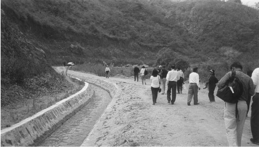
Plate 3.23 UNODC funded water viaduct for rice fields – Mong Ka.
