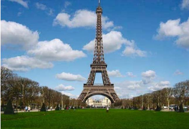
**Fig. 9.14.** The great Eiffel Tower, Paris (1889), was designed by the famous French engineer Alexandre Gustave Eiffel. Built with 7,000 tons of wrought iron to make the perfect geometrical structure having total height of 320 meters
