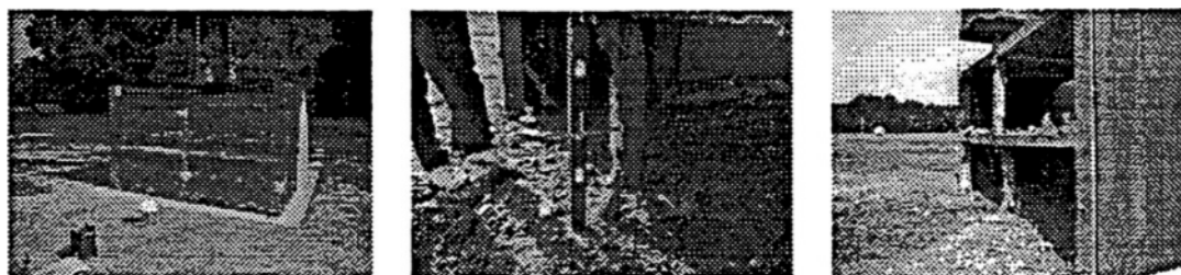
Figure 4: In-Fill Walls, Severe Damage to Column
