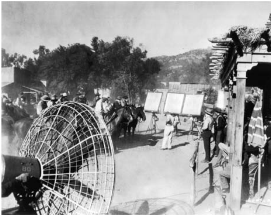
Figure 12.8 Most physical effects are the result of special effects crews using machines and chemicals to produce atmospheres and environments critical to the production, such as the Paramount crew on this Western set preparing to create wind. (Courtesy of Paramount Pictures.)
