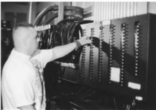
Figure 6.10A and B Light control patch bays may be designed to require physically placing patch cords into patch panels ( left ) or all connections can be performed through a computer program and computer-controlled distributor systems ( below ). (Courtesy of Colortran.)
