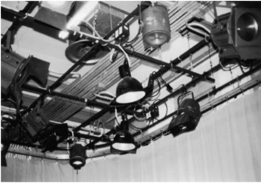
FIGURE 6.7 The lighting grid in a studio is constructed to support both the batten, which carries the power to the pigtails, and the lighting instruments. The grid must be high enough to allow wide-angle shots, but it also must allow for space above the grid to dissipate the heat generated by the lighting instruments.
