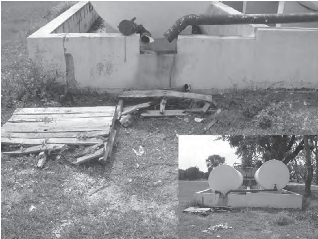
Figure 6.10 Exterior observations—Storage tanks (insert) with evidence of release (provided by Derrek Verlaan).
