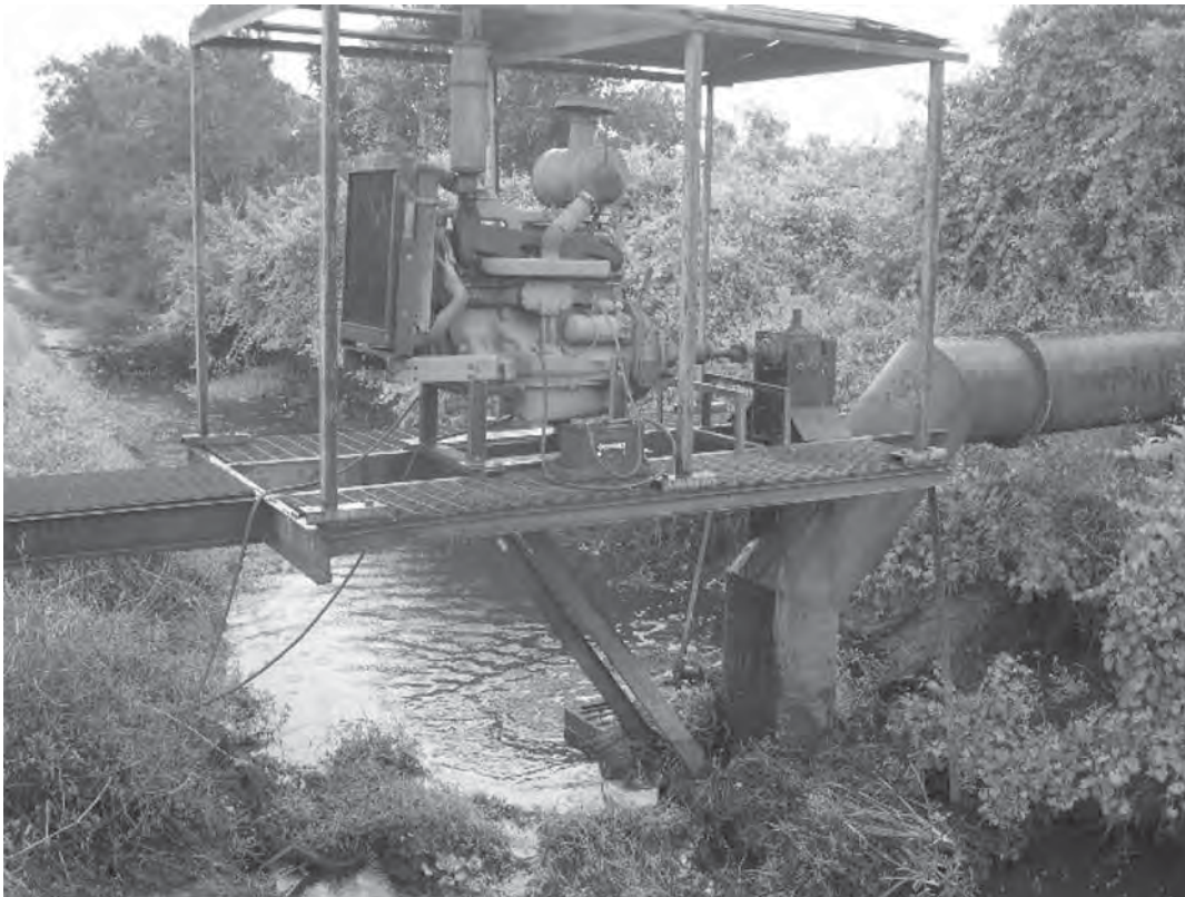
Figure 6.13 Diesel pump with unprotected fuel lines causing release to the canal below (provided by Derrek Verlaan).
