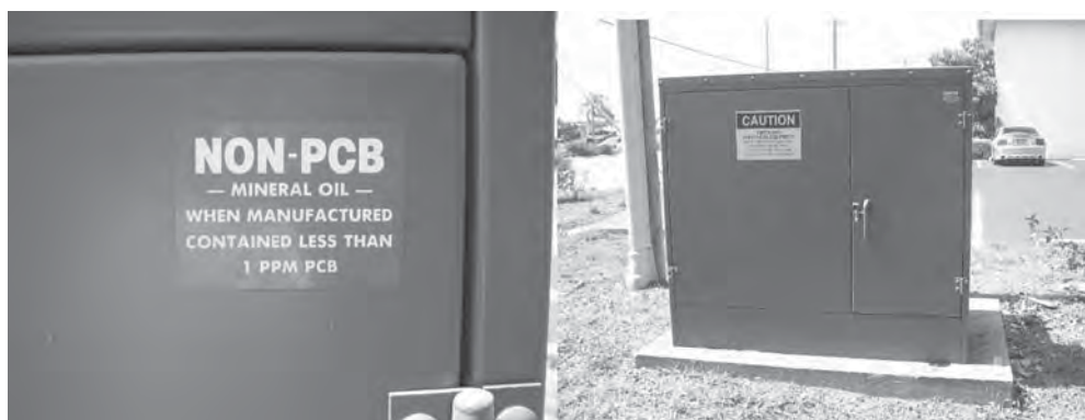
Figure 6.21 Documenting transformer and oil label (provided by Derrek Verlaan).
