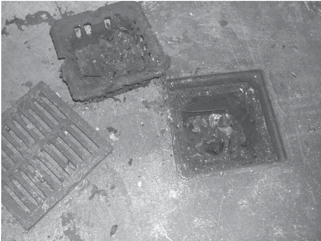
Figure 6.12 Interior observations of a floor drain with a solids trap (provided by Derrek Verlaan).
