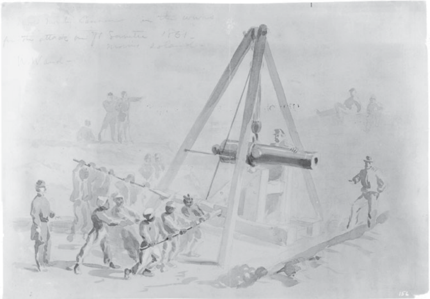
A team of black laborers mounting cannon in the works for the attack on Fort Sumter, March, 1861. (The Library of Congress)
